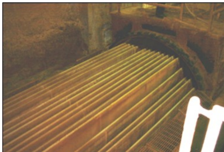
Figure 3. Typical Kelly filter used for the test.
